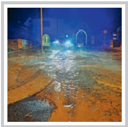
Wasserrohrbruch in Kemnath
